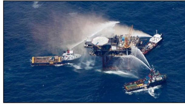
Figure 2.2-1- External fire-fighting operation.
